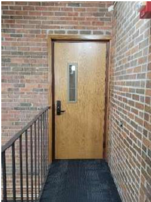
Mezzanine access from elevator
