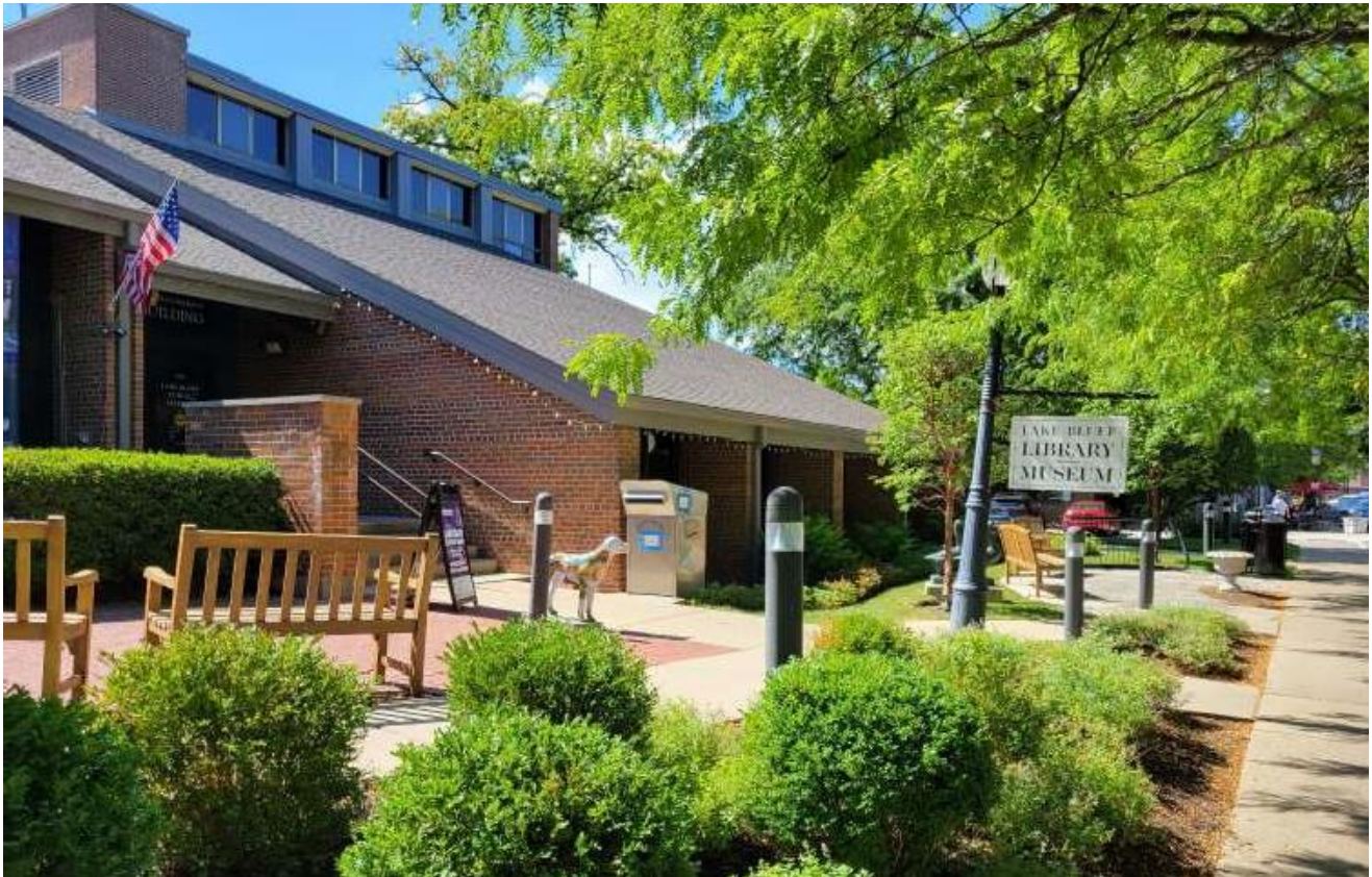
Library Main entry looking west
