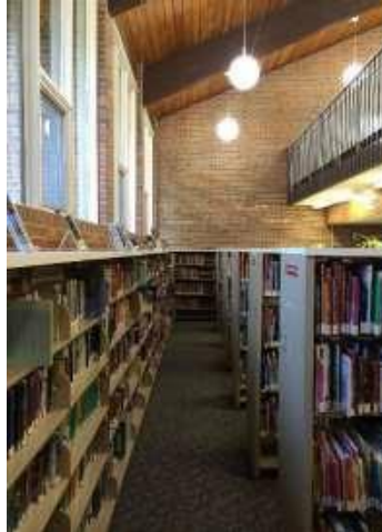
Open Mezzanine edge above Youth Services
