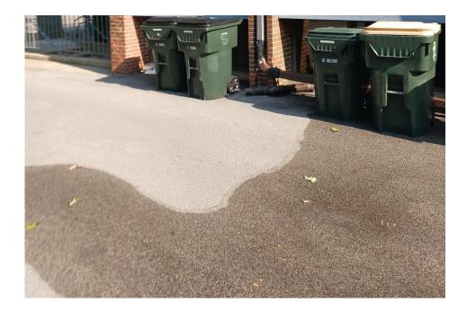
The site's sidewalks show significant signs of wear. The western walk from the Scranton Avenue sidewalk to the doorways has differential settlement, is old and pitted. To eliminate the bumps created by the differential settlement, edges of the sidewalk have been ground down. Gaps are present between sections of the sidewalk. Additional gapping is present by the stairs to the west of the walk. The concrete stairs are worn. The hand railing seems insufficient.
