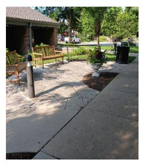
The looping ramp located at the front of the property appears to be ADA compliant, although a survey is required to verify. The eastern portion of the ramp is undermined, with the bottom exposed. This should be backfilled / mud-jacked to avoid future issues. The intersection with the public walk and the main walkway appears to have a greater than 2% slope and is not ADA compliant. The public walk would need to be adjusted to address this issue.
