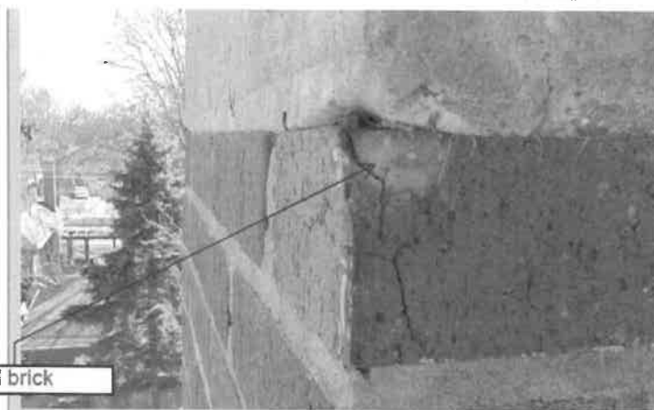
Gap at Beam support, concrete
