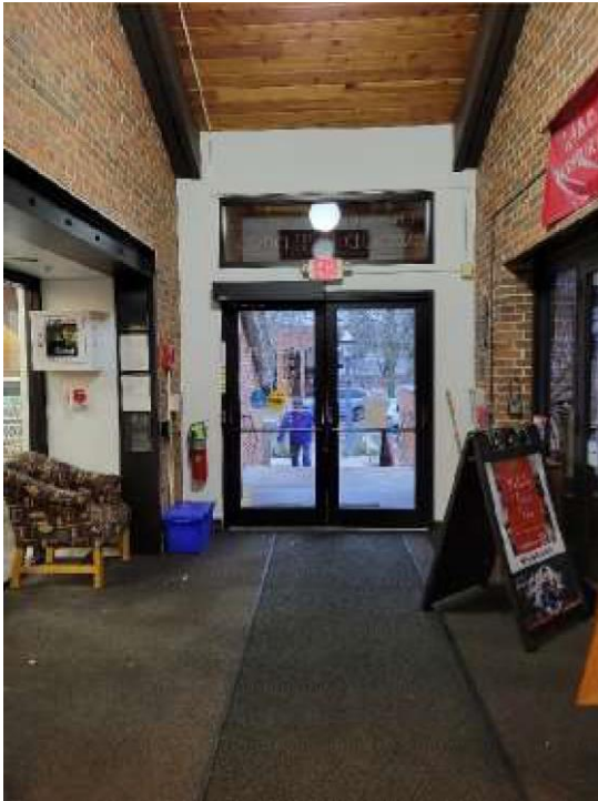
Library Entry looking toward Elevator
